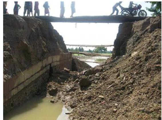
Damaged culverts and bridges in the Far West
